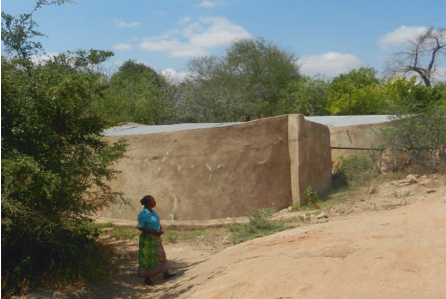
Fig. 4 Miamba Mitamboni water storage tanks with the native acacia woodland in the background, southern Makueni County. (Photo by author 2013)
