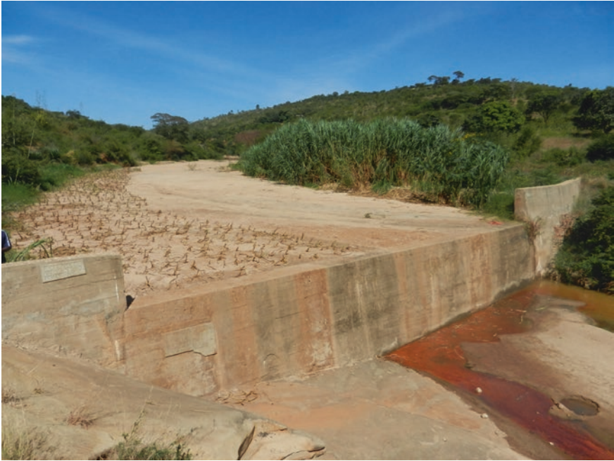
Fig. 5 This sand dam was built in 2009 by the Kitandi Fruit Tree Growers SHG on the Kaiti River in northern Makueni County. It was extended 1 year later to reach its present height. It has a 17.9 meter spillway and holds nearly 11,000 cubic meters of sand and 4000 cubic meters of water when saturated. Note the strong stand of napier grass on the right stream bank. It is also planted as cuttings on the left bank. (Photo by the author, July 2013)
