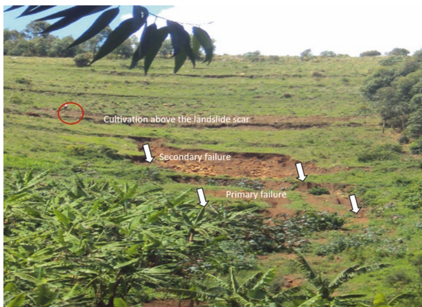
Fig. 12 Landslide reactivation due to cultivation around the landslide scars, 2016. (Photo credit: Nseka)
