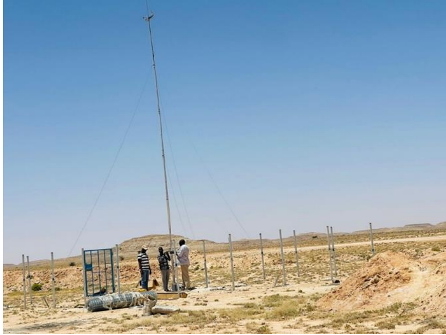
Badhan Airport station
